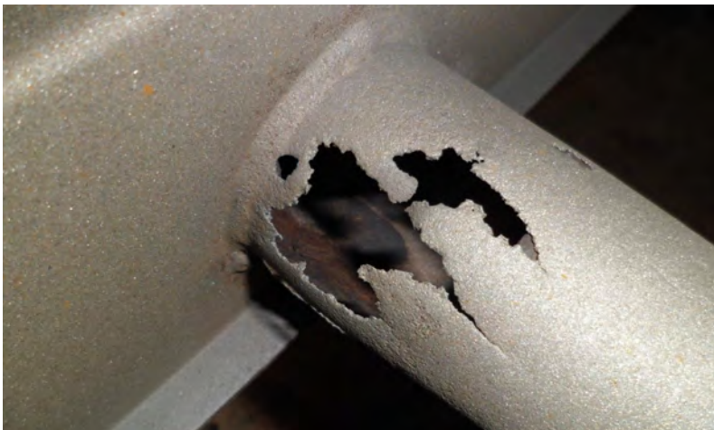
The original hole had gotten somewhat larger since blasting (as expected)
