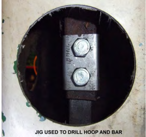
JIG USED TO DRILL HOOP AND BAR
