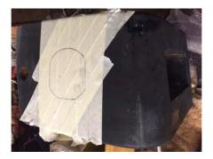
Now check the socket fits. It might need minor trimming to make it fit. Holding the socket in, use a small drill bit (roughly 2.5mm) and drill the 4 retaining screw holes and pop in some screws. I used stainless steel as being on the outside of the Fox, if I need to remove it, hopefully they won't have rotted away!
