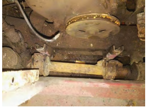
Looking down from above, before the fresh rack was fitted.
